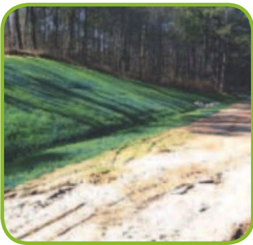
Turf Reinforcement Mat with three weeks vegetative establishment.
