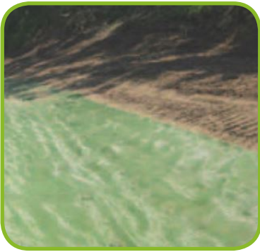
Second generation woven turf reinforcement matting used for steep slope channel stabilization.
