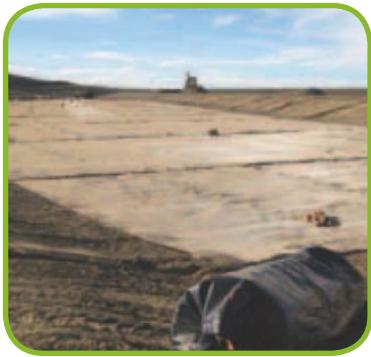
High-Performance turf reinforcement mat with superior ultra-violet resistance for up to a 50-year design life in semi-arid conditions.
