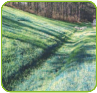
First generation turf reinforcement mat used for channel stabilization.
